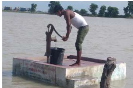
Raised latrines, boat for rescue and handpump on elevated platforms as local flood risk reduction efforts.
